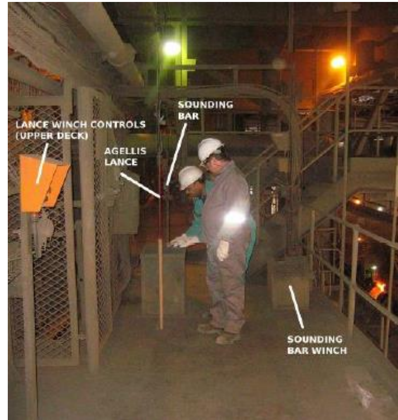
Figure: Sounding bar at Vale
