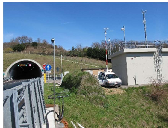
Figure 1. “Direct RF radiation” with antennas positioned outside gallery’s entrance.
