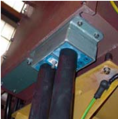
Installations of Roxtec sealings
